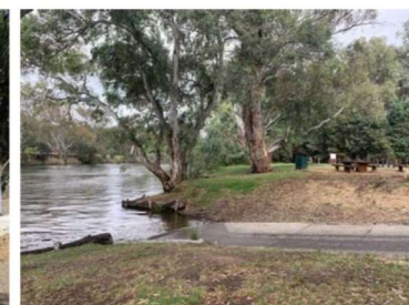
Concrete boat ramp and adjacent picnic area.
