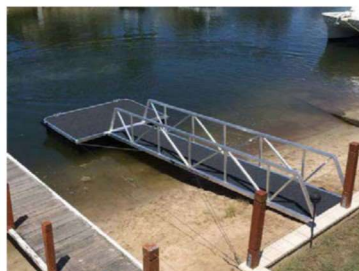
Floating pontoon jetty.
