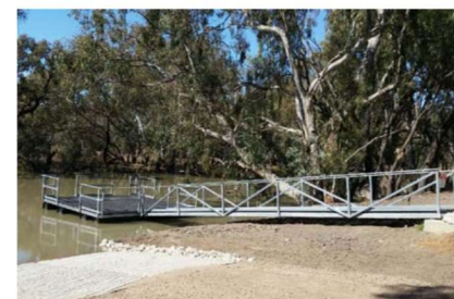
Floating pontoon jetty.
